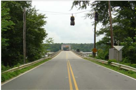
Shoulder Widths less than current standards
