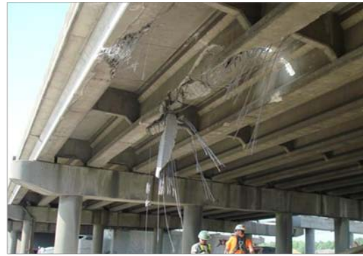
Vertical underclearance less than current standards
