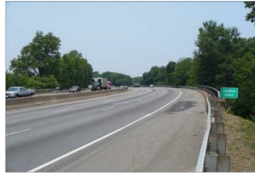
Shoulder Widths less than current standards
