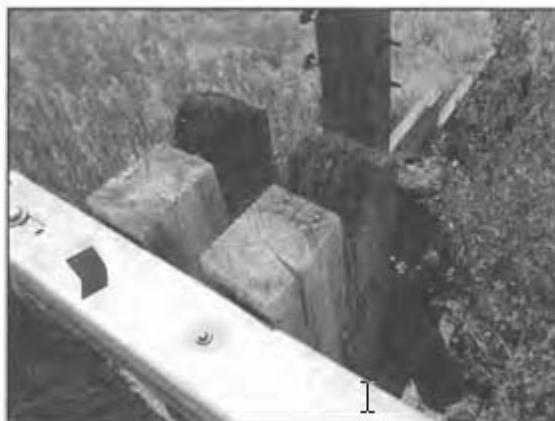
Figure B-5-Decay in Timber Rail Posts
