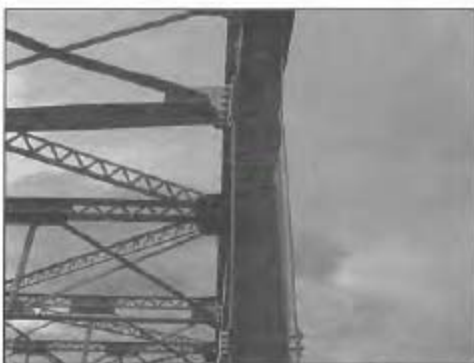
Figure B-15—Sway Bracing Impact Damage in Span 1
