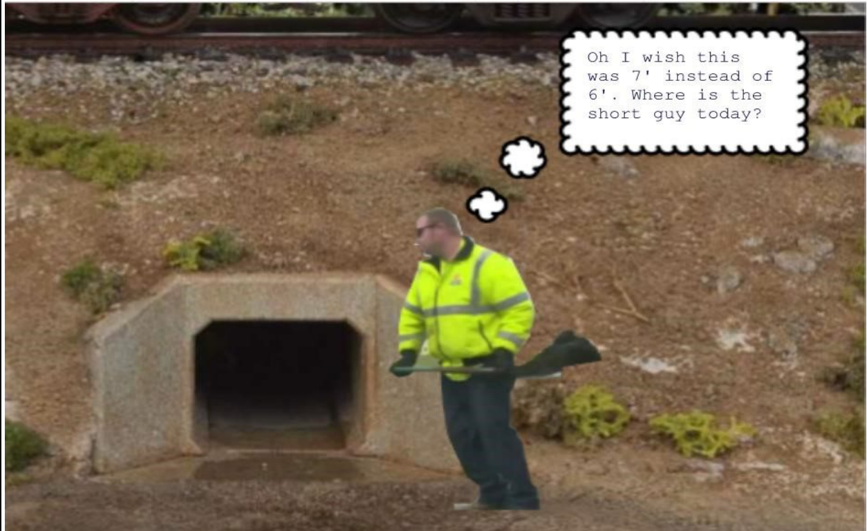
6' tall culverts attempting to be cleaned
