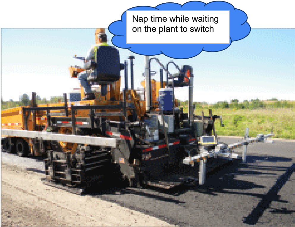
Paving the 0.75 ASPH BASE layer
