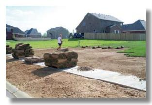
Sod reduces erosion potential to near zero. Make sure the surface is properly prepared with appropriate soil amendments; use fresh sod and keep well watered during the first 2 weeks after application.
