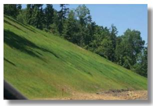
Establishing grass through broadcast or hydro-seeding reduces erosion and sediment loss by more than 90 percent. Use mulch on short flatter slopes and erosion control blankets or hydro-mulch on long steep slopes.
