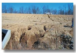
Long, bare slopes need to be stabilized. Polyacrylamide offers excellent temporary protection for slopes that will not be seeded or mulched immediately. Do not use near creeks, rivers, or wetlands. Follow manufacturer's instructions.
