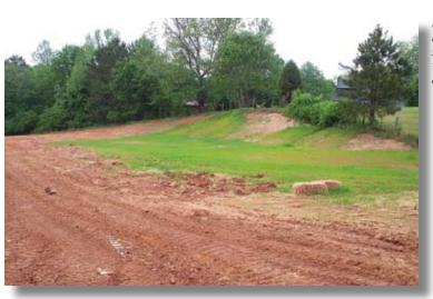
Designate haul roads and material storage areas on large sites, and seed or mulch the rest to minimize the amount of bare areas exposed to the weather.
