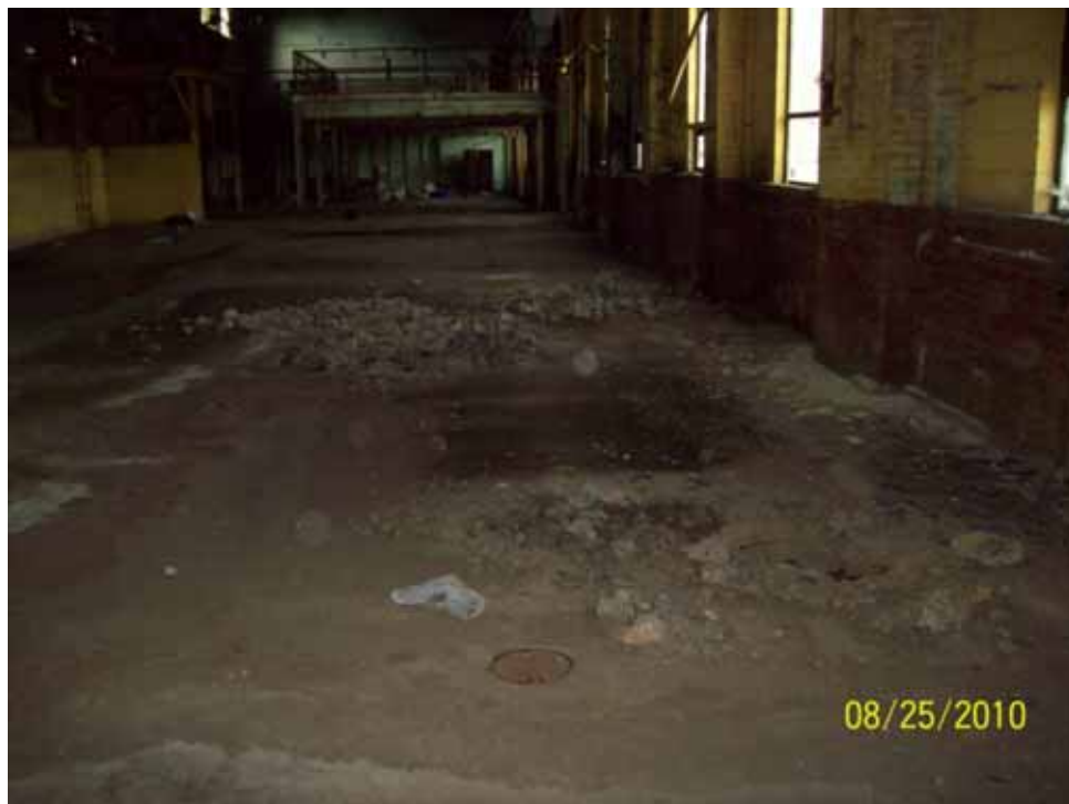
PHOTO 12: View of east end of Main Street Building (East Main Plater area) looking from the east wall west. Monitoring well W-3 in foreground. Broken concrete represents general locations of 1997 sampling locations EMP-6 through EMP-9 and 1999 location BW-5.
