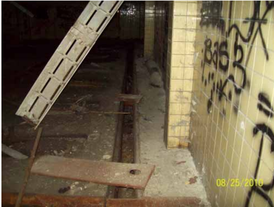
PHOTO 7: View looking south from north end of East Shop, of floor trench running along the west wall of the East Shop. Note debris and overhead obstacles throughout the East Shop.
