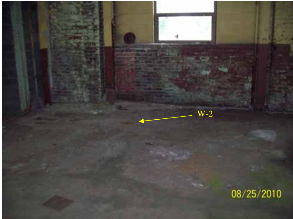
PHOTO 11: View of monitoring well W-2 near north wall Main Street Building.
