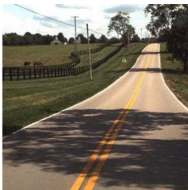
Typical RS Pavement
